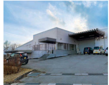
The Tsumagoi Meisui Co. Ltd production plant
